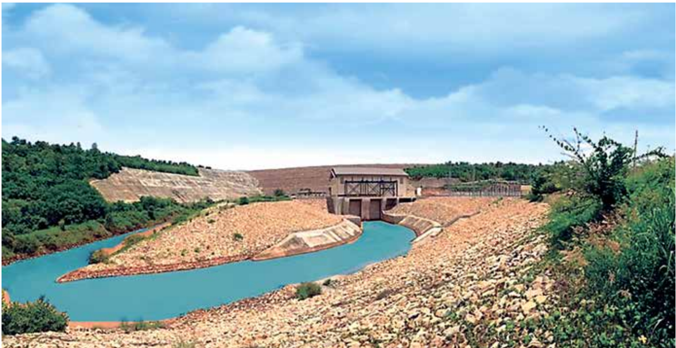
Pasak Jolasid Hydropower Plant
