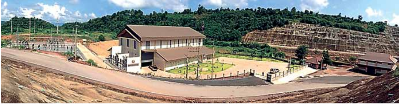
Khwae Noi Bamrungdan Hydropower Plant
